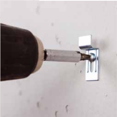
Fixing for the wall that holds the Panel hanging system.
